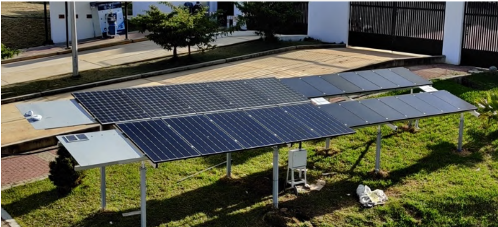
Fig. 4.1 Top view, at the bottom left is the PERC array under analysis at Chachapoyas.
