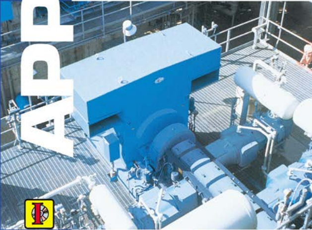
Synchronous motor 2500 HP at 327 RPM with WPII enclosure driving a reciprocating compressor in a refinery.
