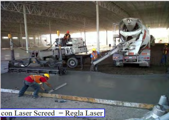
Concrete floor leveling with Laser Screed
