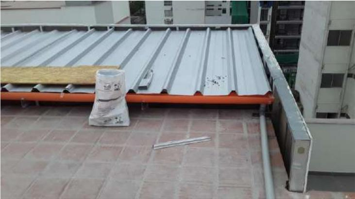
A photograph showing a section of a roof under construction. A corrugated metal sheet (TR-4) is laid out on a wooden frame. A white bag of material and a metal rod are placed on the roof surface. The background shows a building with windows. |
