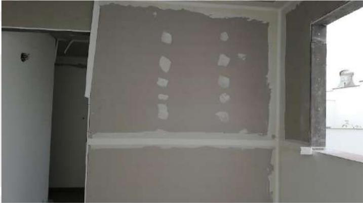
A photograph of an interior wall during renovation. The wall is covered with a grey joint compound, and white tape is applied to the joints between the panels. A window is visible on the right side of the frame.                              |
