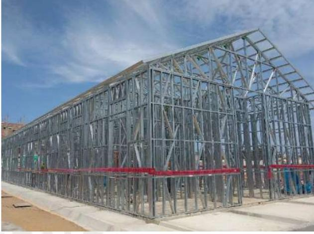
A wide-angle photograph showing the exterior of a large industrial building's steel skeleton. The structure consists of a grid of vertical columns and horizontal beams, with a pitched roof structure. Red safety tape is strung across the lower part of the frame. The ground is a mix of dirt and concrete. |
