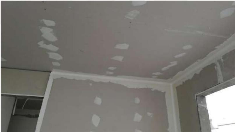
A photograph of an interior ceiling during renovation. The ceiling is covered with a grey joint compound, and white tape is applied to the joints between the panels. A window is visible on the right side of the frame.                       |
