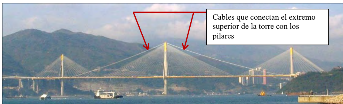
Figura 3.4-4: Puente Ting Kau ( https://en.wikipedia.org/wiki/Ting_Kau_Bridge ).
