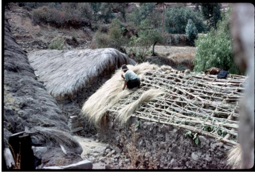
Figure 38. Ichu thatch being tied to roof in Peru in 1970.
