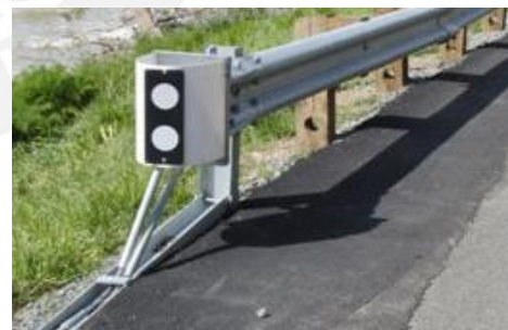
Fig. 3.31: Terminal X-Tension
