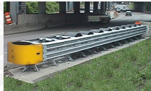
Fig. 3.53: QuadGuard Elite Fuente: Energy Absorption Systems, Inc.
