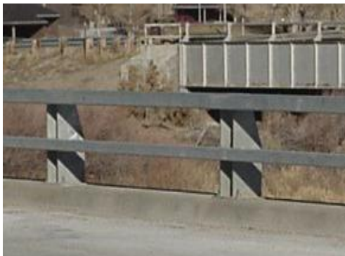
Fig. 3.23: Wyoming Two-Tube Fuente: FHWA
