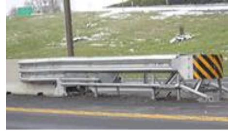
Fig. 3.49: QUEST Fuente: Energy Absorption Systems, Inc.
