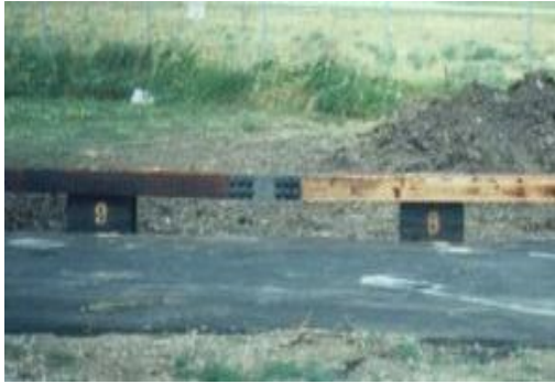
Fig. 3.21: Curb type glu-lam timber railing Fuente: FHWA
