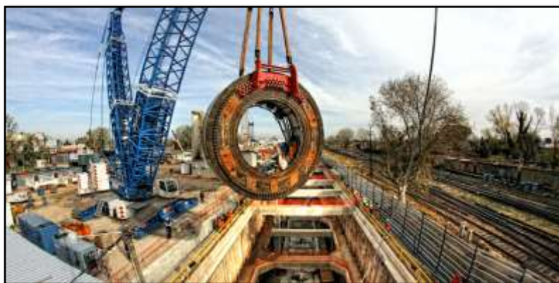
Figura 2: Montaje de TBM [3]
