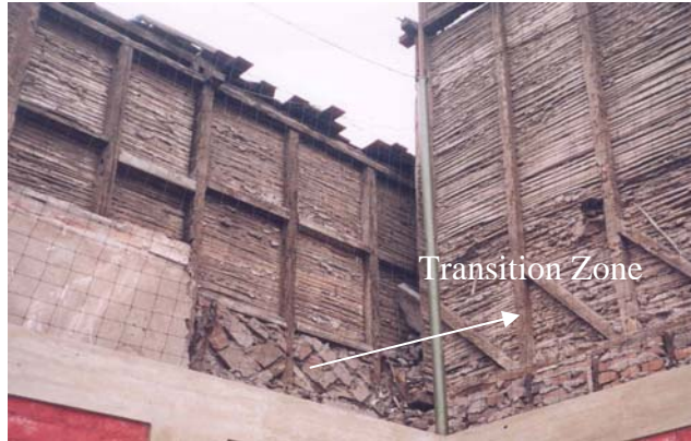
Transition zone construction
