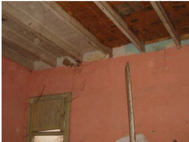
Typical roof structure
