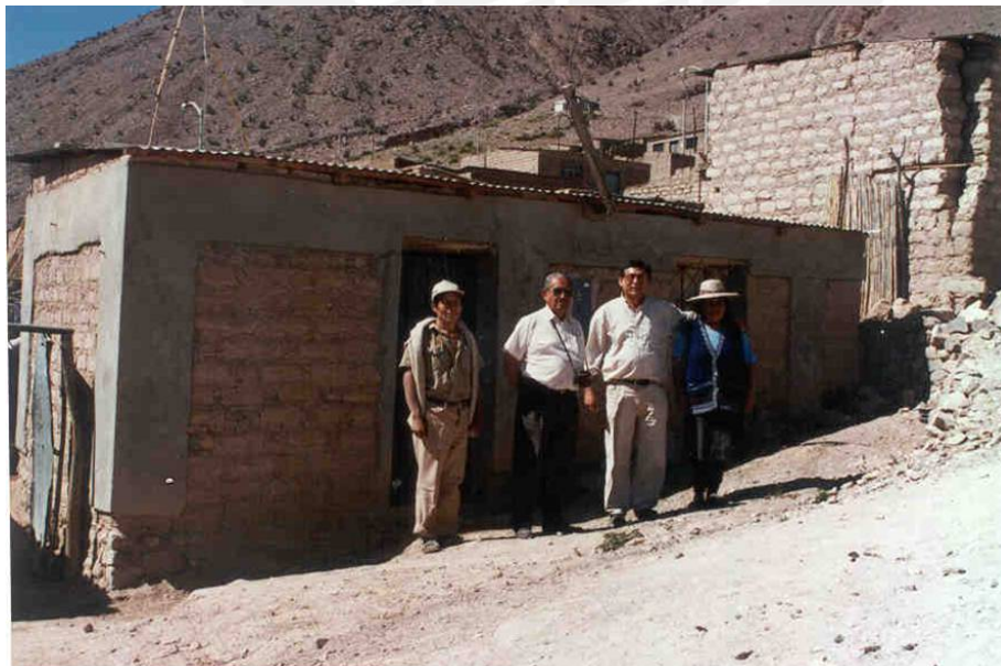
House retrofitted with wire mesh after an earthquake without damage, neighbor's house collapsed (photograph by San Bartolomé 2002)
