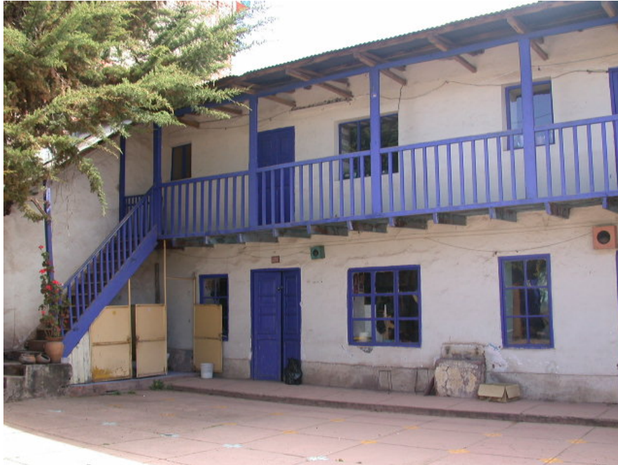
Means of escape: each room has its own door.
