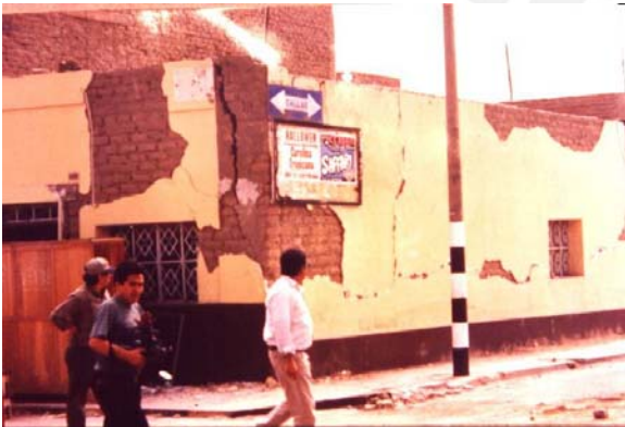
Damage on corners by Traction – flectional strength (photograph by San Bartolomé 2002)
