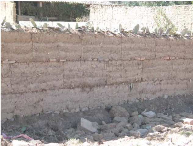
Left: Wrong construction practice (mixture of soil with gravel and without straw). Right: Well construction practice (mixture of soil and straw, uniform compactation)
