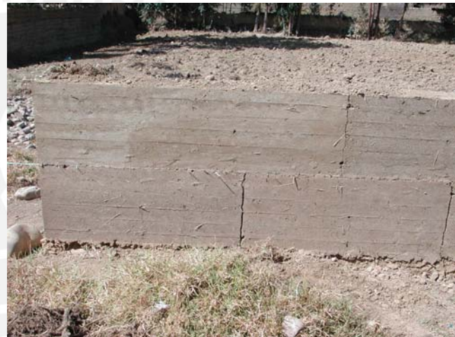
Left: Wrong construction practice (mixture of soil with gravel and without straw). Right: Well construction practice (mixture of soil and straw, uniform compactation)
