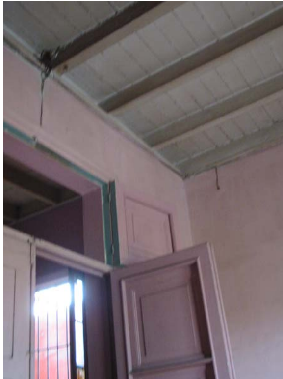
Typical roof system in republican buildings
