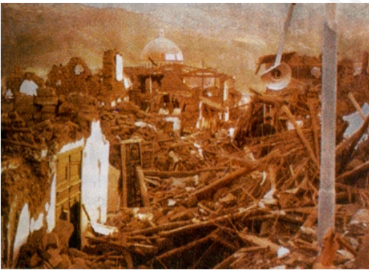
Huaraz city: 100% adobe buildings destroyed during 1970's earthquake (Kuroiwa 2002)
