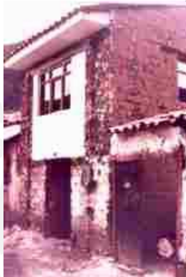
Seismic strengthening technologies: Retrofit with wire mesh. Retrofit of adobe contemporary house (photograph by San Bartolomé 2002)
