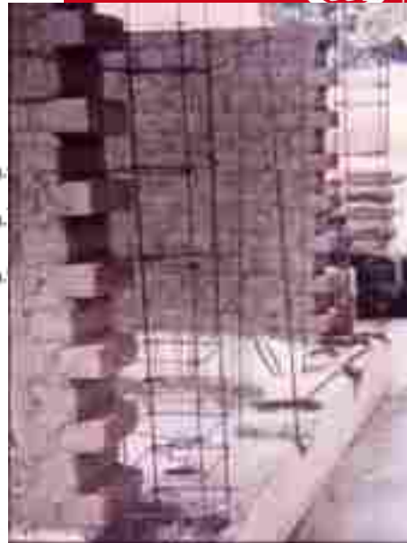
Seismic strengthening of new construction: Spandrel wall retrofitted with timber planks (left).
