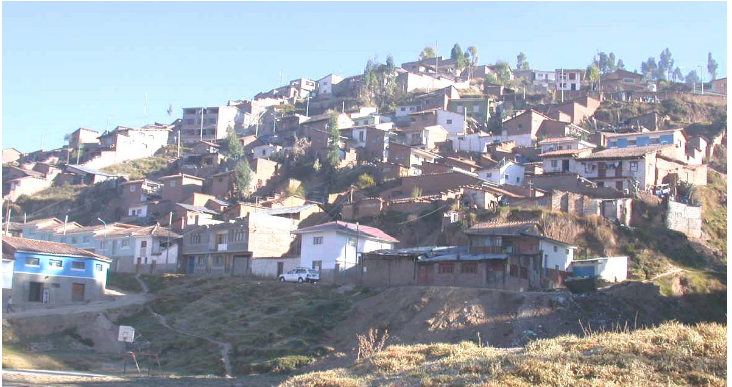
Adobe house building on Cusco hills
