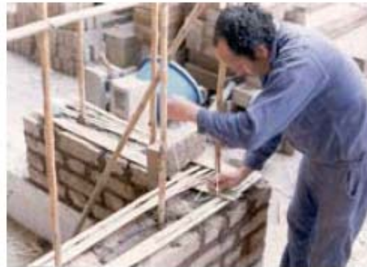
Seismic strengthening of new construction: wall Reinforcement with canes (MTC 2000)
