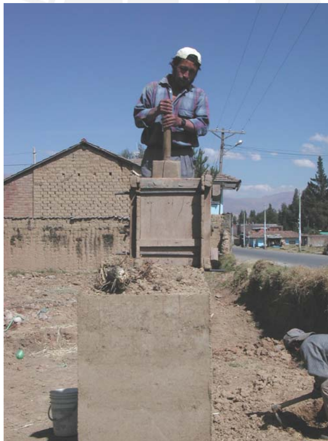
Tapial wall construction
