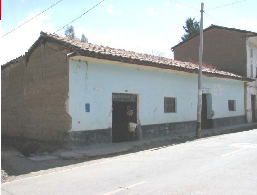
Typical tapial house with gable roof
