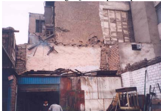
Typical Problems in These constructions: humidity and non maintenance. The wood is attacked by insect, the walls are destroyed.
