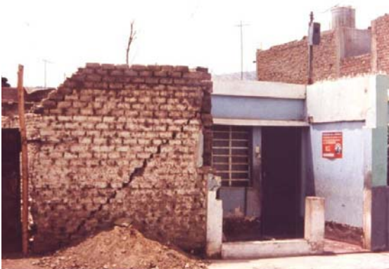
Damage by diagonal traction strength (photograph by San Bartolomé 2002)
