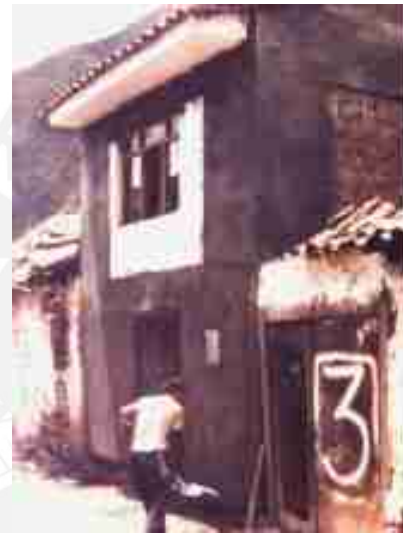
Seismic strengthening technologies: Retrofit with wire mesh. Retrofit of adobe contemporary house (photograph by San Bartolomé 2002)
