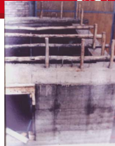
New Construction of Tapial Walls with vertical and horizontal canes. Walls joined by a concrete beam. (photograph by San Bartolomé 2002)
