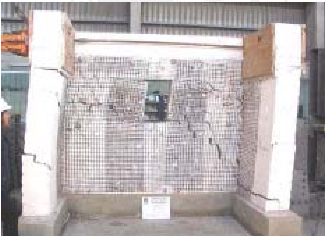
Adobe wall reinforced with geosynthetic after seismic test (Madueño 2005)
