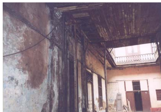
Typical Problems in These constructions: humidity and non maintenance. The wood is attacked by insect, the walls are destroyed.
