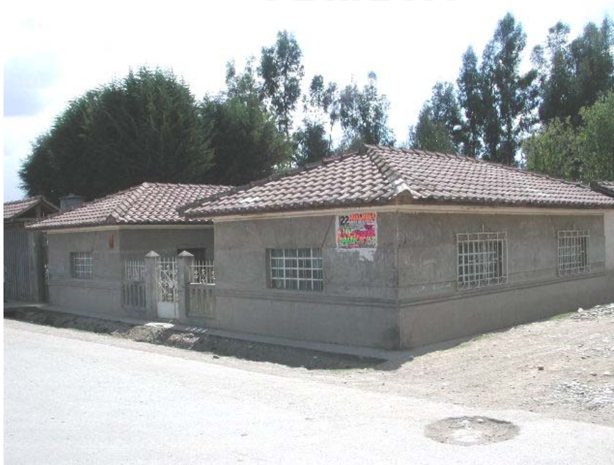
Tapial house with hip roof
