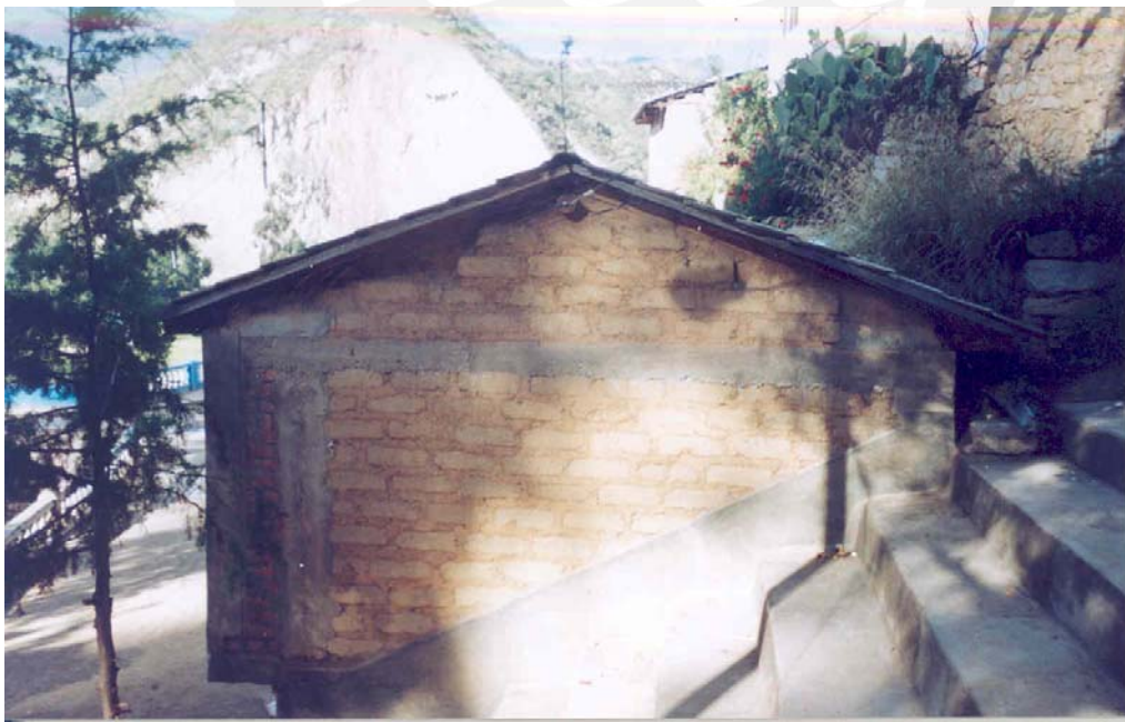
New house construction with wire mesh and concrete beam
