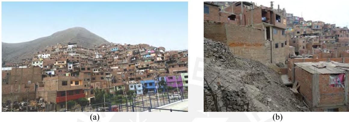
Figure 1. Informal and disorderly construction of confined masonry dwellings in Lima-Peru (Sato, 2018)
