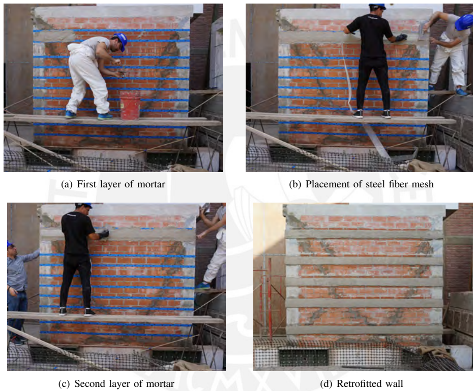
Figure 6. Stages for strengthening CMW with SRG (W-02)
