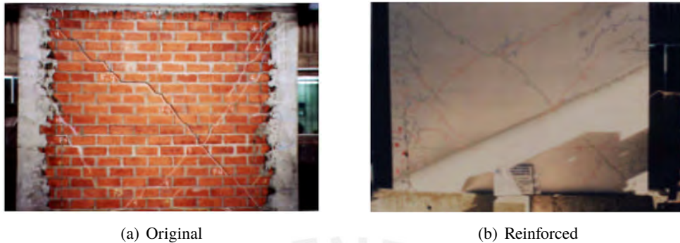
Fig. 5 Strengthening with welded mesh WM
