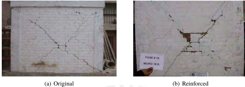
Fig. 7 Strengthening with GFRP
