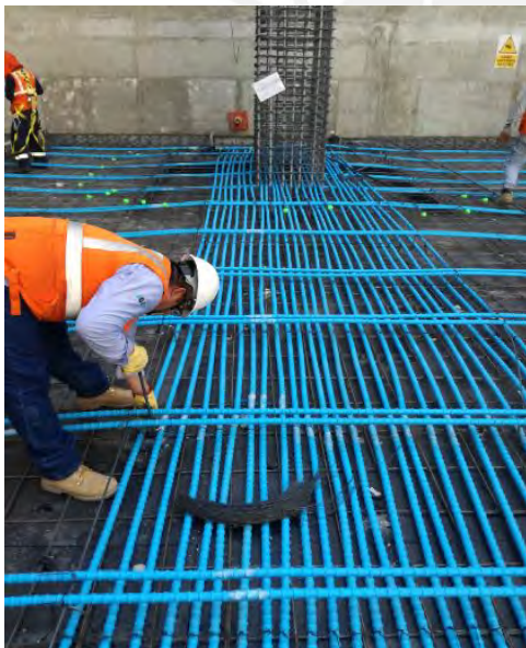
(a) Vista general de amarre.
