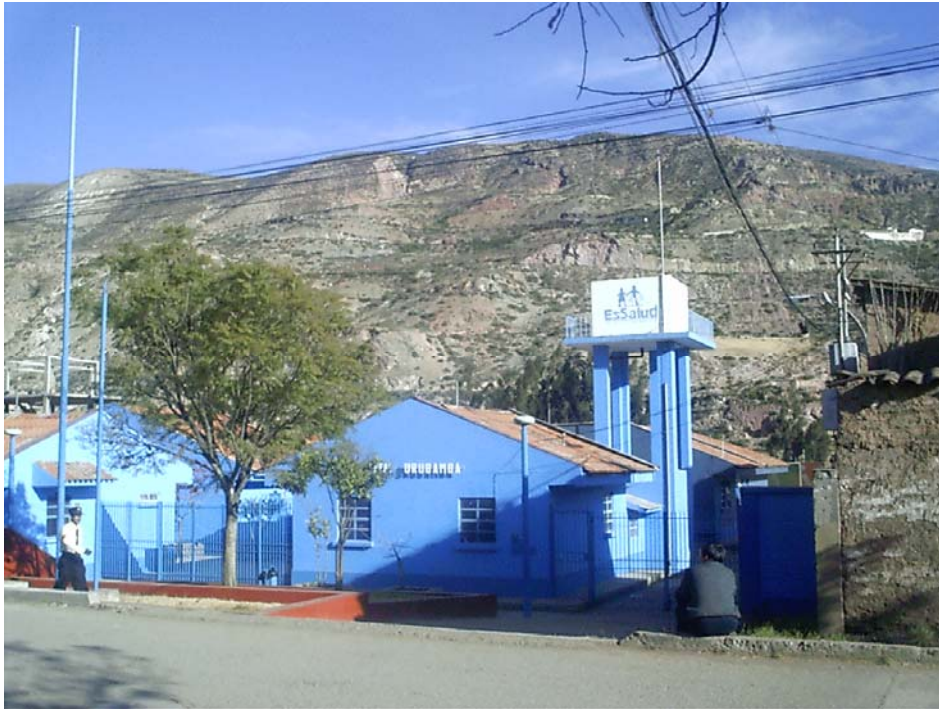
Figura 1.2 Hospital ESSALUD de Urubamba
