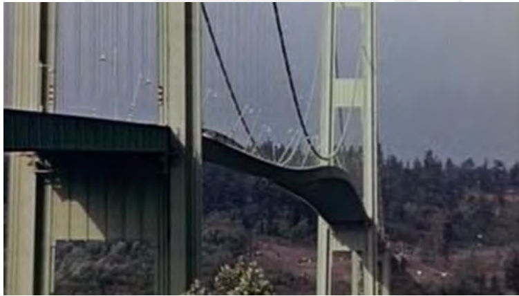
Figure 3.1: Collapse of the Tacoma Narrows Bridge in Washington [33]
