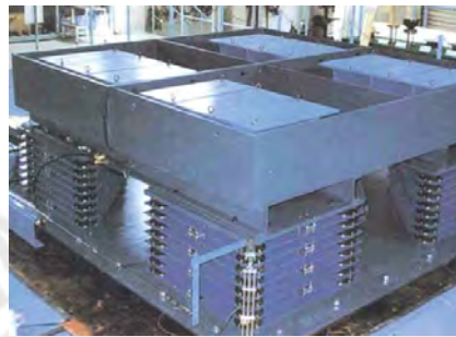
Figura 1-7 Tuned mass damper for Chiba-Port Tower (Connor & Laflamme, 2014)
