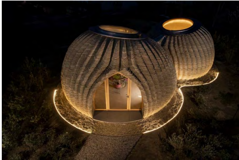
Figure 2.5. 3D printed clay house (Mario Cucinella Architects, 2024)
