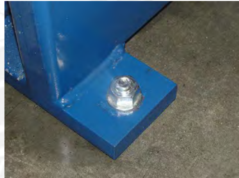
Anchor Bolts in position.
