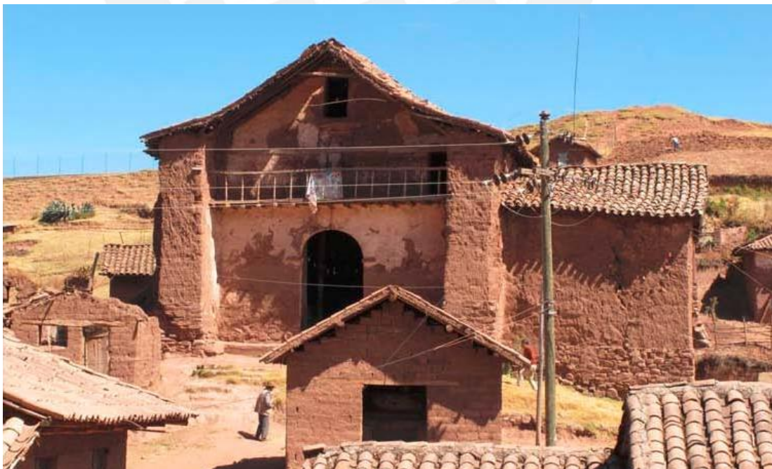
Fig. 30- Fachada principal (extremo sur) [1]
