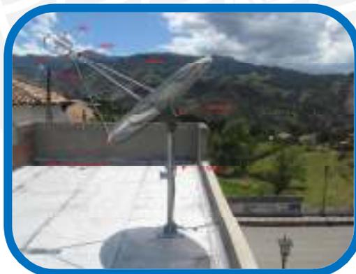
Figura 2 Antena Satelital Instalada
