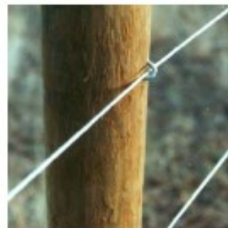
Figure 1 Loose Stapling of Fence Wire
