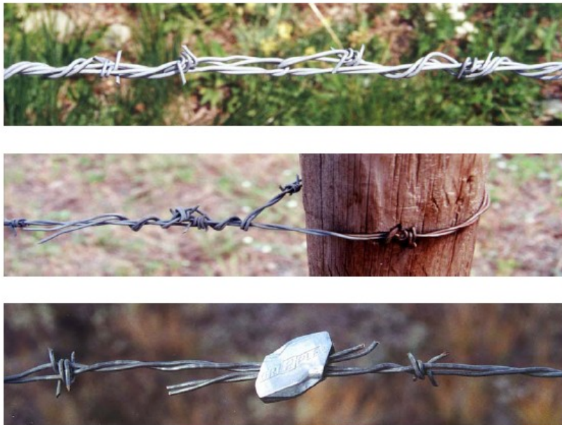
Figure 4 Knots and Mechanical Splice for Barbed Wire
