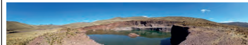
20220514_LAMPA_COMPUERTA_CE_019 LAT. 15°42'36.5"S, LONG. 70°36'29.1"O
