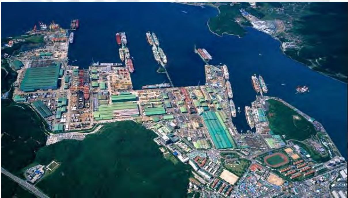
Figura 59. Samsung Heavy Industry shipyard. Tomado de “Shipbuilding,” por Maritime Connector, 2011. Recuperado de http://maritime-connector.com/wiki/shipbuilding/
