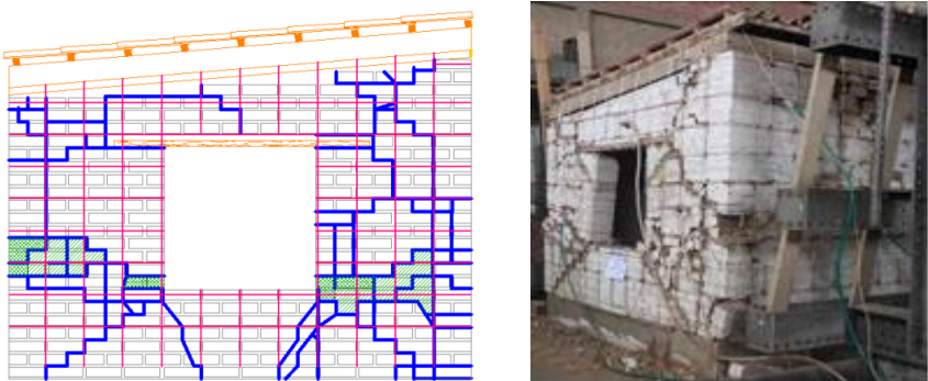
Fig. 2. Sketch of damage pattern and general view of the model after shaking table testing.
