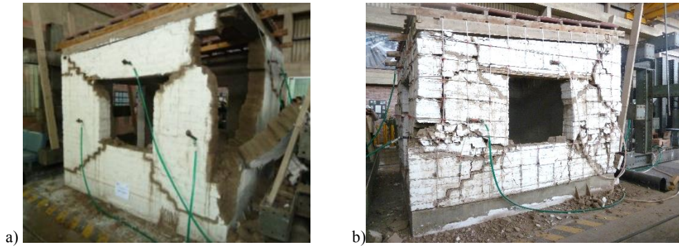
Figure 1. Sketch of damage pattern and general view of the model after shaking table testing.
