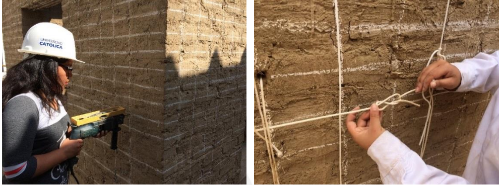
Fig. 6 Reinforcement process. Left: drilling crosstie holes. Right: tying the horizontal ropes
